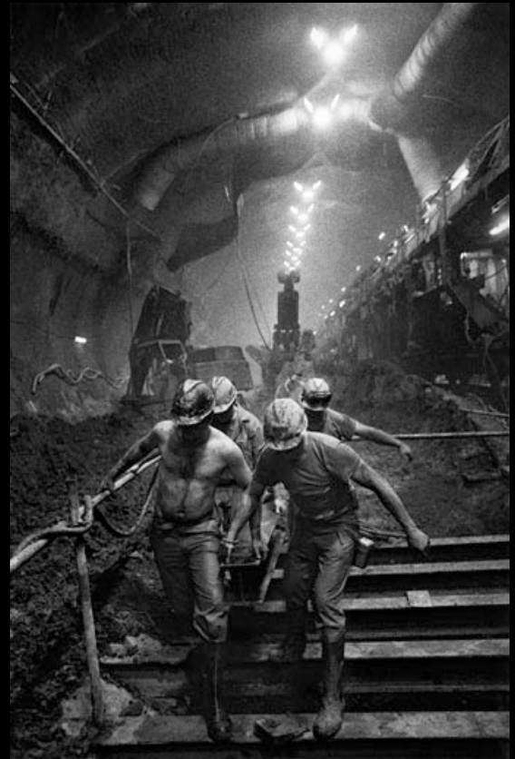
(21) Works of the tunnel under the Channel, Folkstone, England, 1990.
