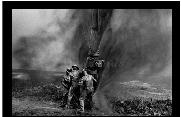
(27) Working on an oil wellhead, Greater Burhan, Kuwait, 1991.
